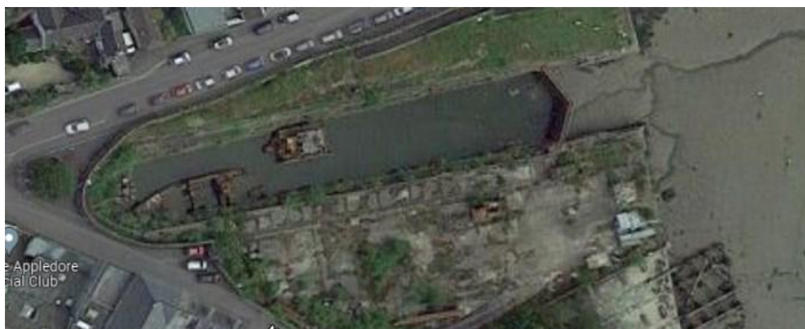
Figure 11: Aerial view of Richmond Dock (extracted from Google Earth, 2022)
