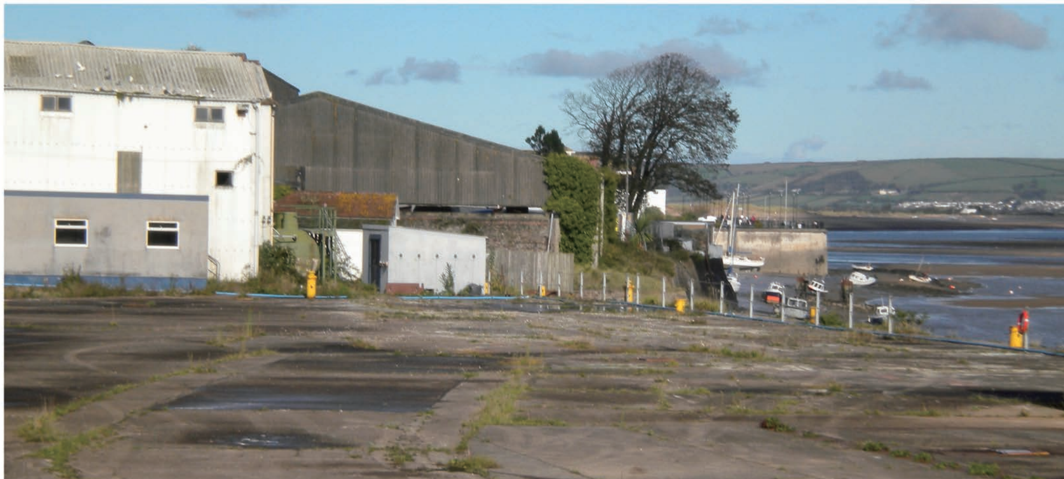
Site of New Quay Dry Dock, Appledore
