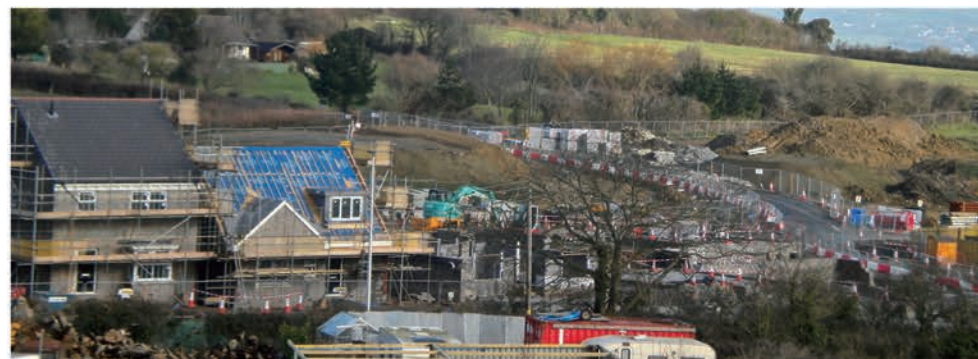
Wooda Road development looking towards Appledore.
